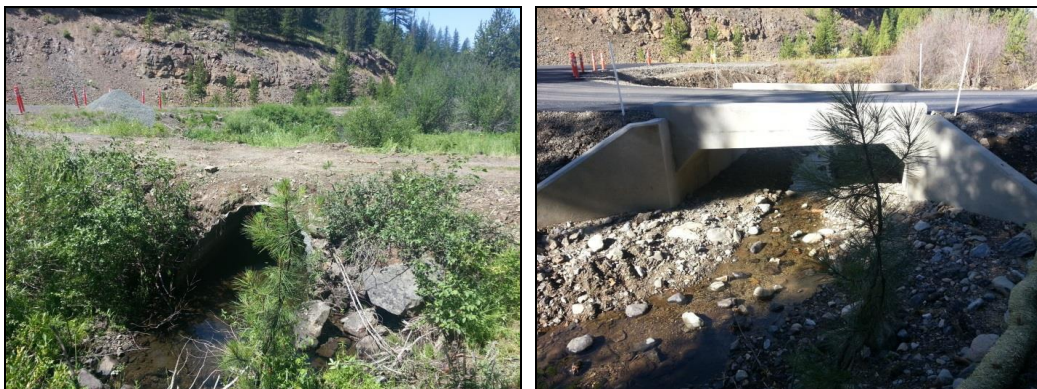
Figure 6. The Bull Run Culvert before replacement (left) and after replacement (right).
