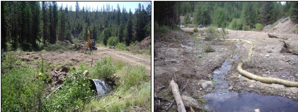
Figure 5. Photographs of the Deep Creek culvert looking downstream before replacement (left) and after replacement (right). Note the ‘after’ photograph was taken from where the old culvert was located showing the meanders created and the new Deep Creek Culverts relative location (60 meters downstream of the old culvert).
